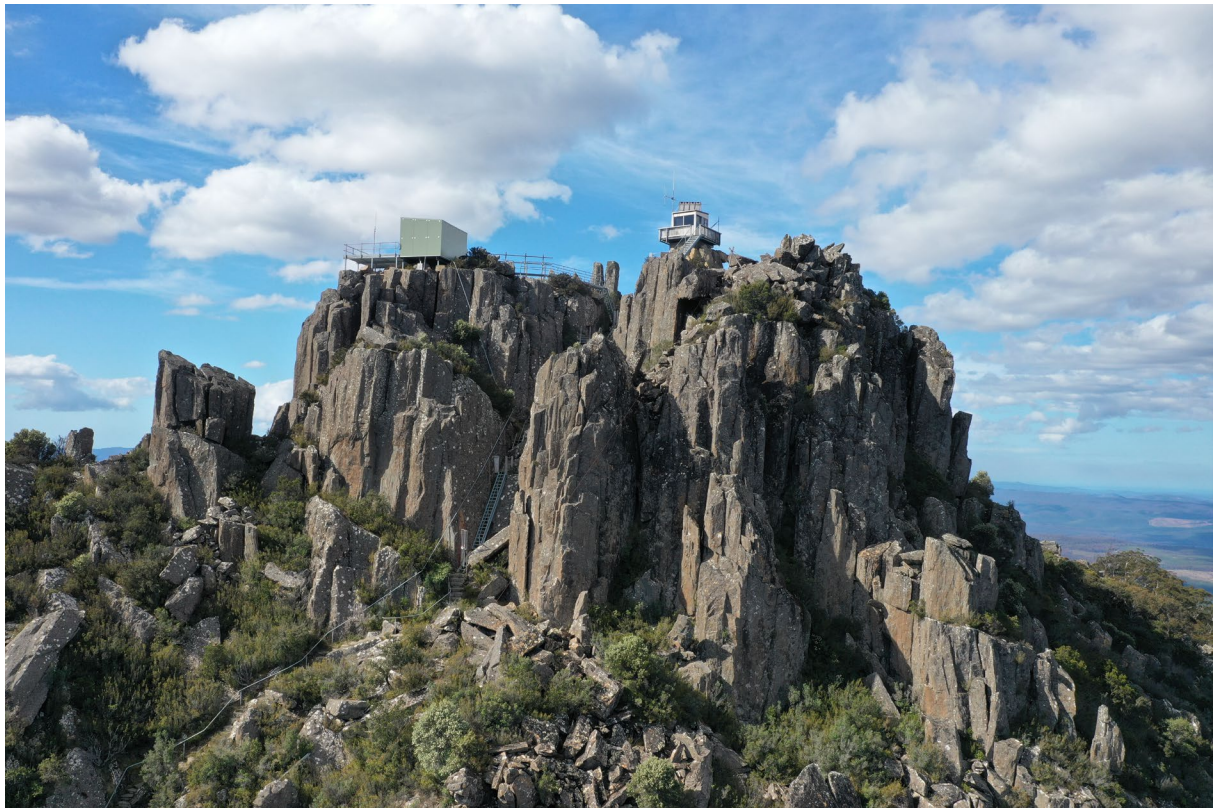
Image: Tower Hill Fire Tower, looking from Fingal
